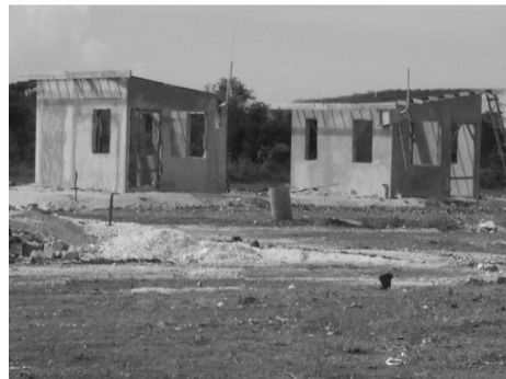
New Housing Construction in Jamaica (left) and Grenada
