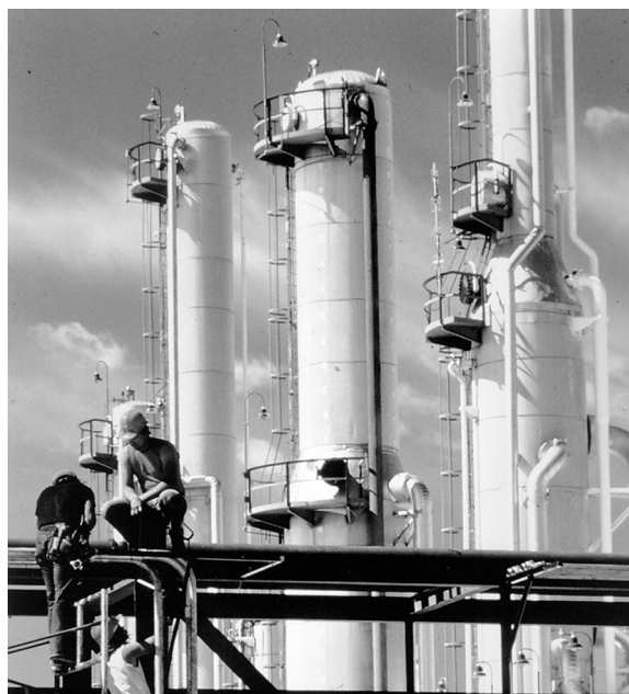
(2) From production wells, gathering lines deliver natural gas to processing plants. Here, natural gas is refined to remove impurities, like water, other gases, and sand.
