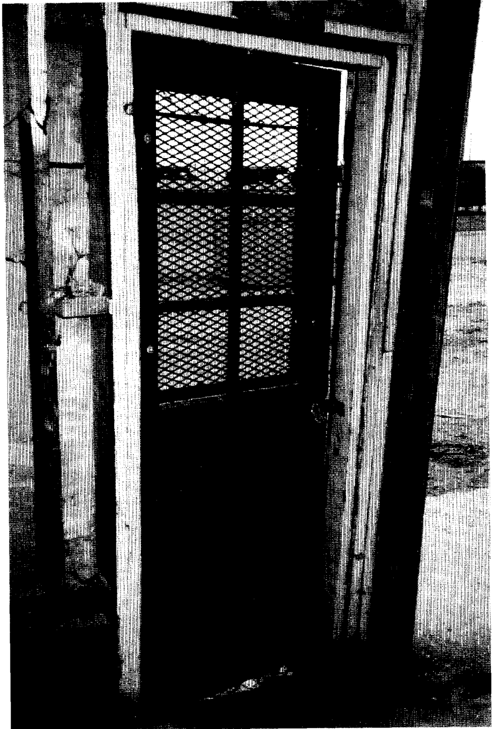
Figure 3.8: Rear Warehouse Door With Unsecured Latch - Fort Campbell
