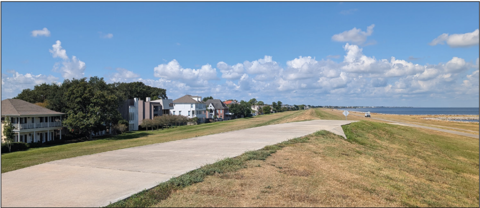
Figure 13: Levee and Protected Homes on Lake Pontchartrain
