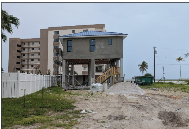
Elevated rebuilt home and vacant lots in Fort Myers Beach (Florida).
