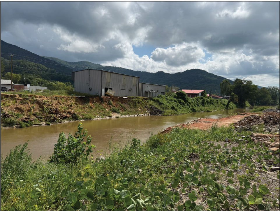
Figure 11: Flood Damage Along the Swannanoa River
