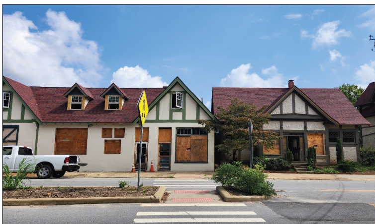
Flood damaged homes in Biltmore Village (North Carolina).
