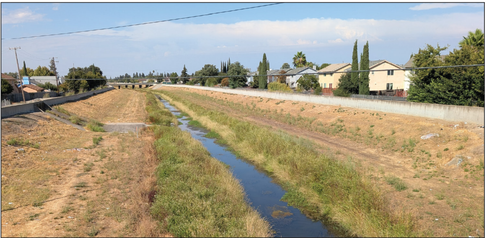
Figure 12: Levee Protecting Homes Along a Canal in Sacramento
