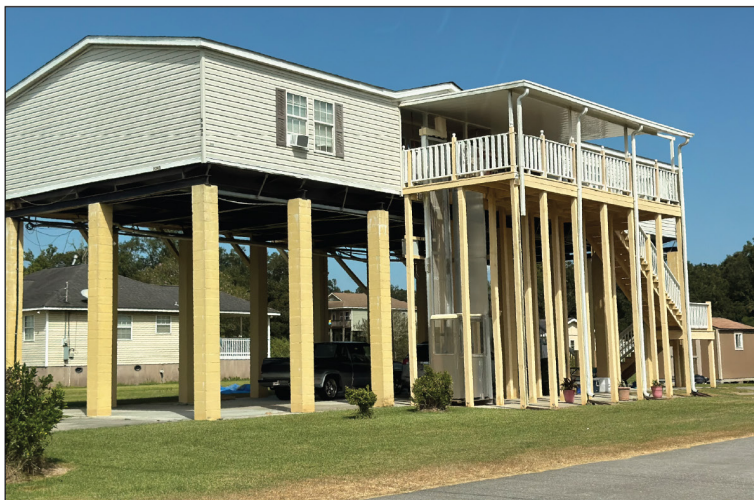
Elevated home across the street from a Mississippi River levee (Louisiana).
