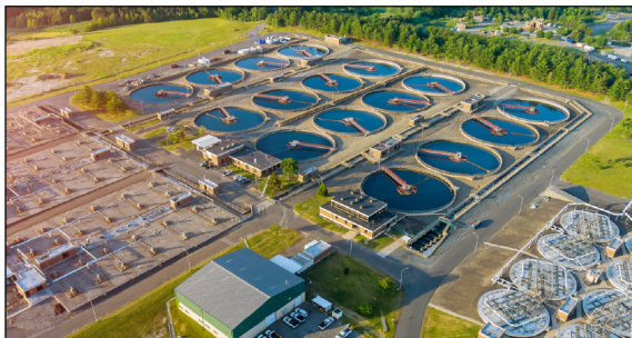
Water systems may contain hundreds of diverse components, making it difficult to properly map and keep operational technologies updated with security patches.
