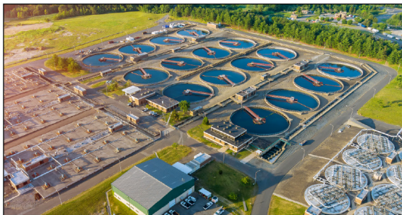
Water systems may contain hundreds of diverse components, making it difficult to properly map and keep operational technologies updated with security patches.
