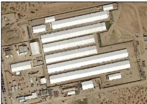
Aerial photo of Camp East Montana
