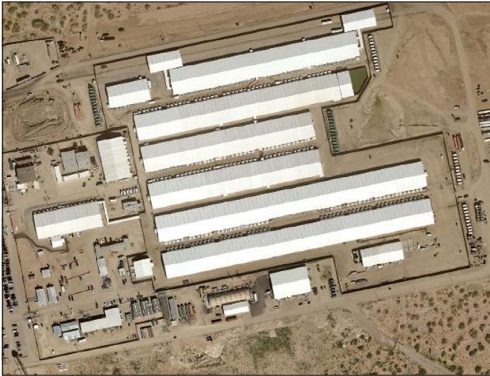
Aerial photo of Camp East Montana
