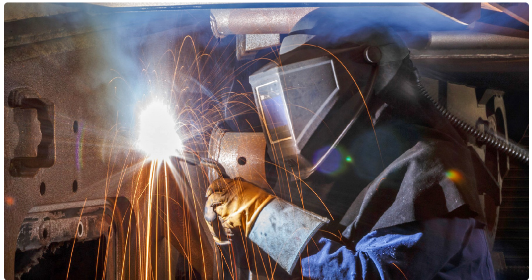
Figure 1: Maintainer Welding at Anniston Army Depot
