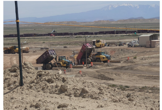
Two trucks unloading containers of tailings at the Crescent Junction Disposal Site.
