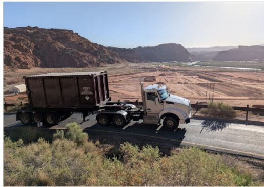
Truck at the Moab Mill Site moving tailings from the pile to the train.
