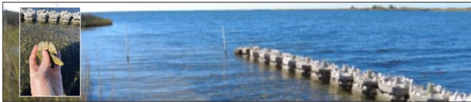
New oyster reefs installed to reduce storm surge damage and slow shoreline erosion. Inset shows young oysters beginning to establish on the reef.
