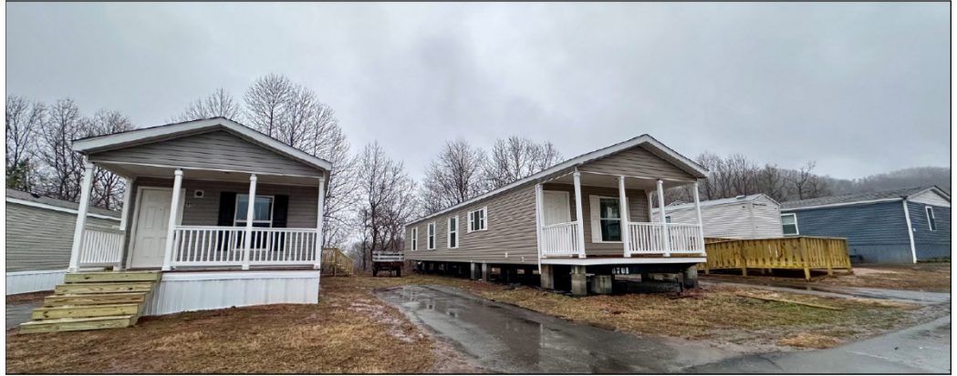
Figure 6: Federal Emergency Management Agency Manufactured Housing Units in North Carolina After Hurricane Helene
