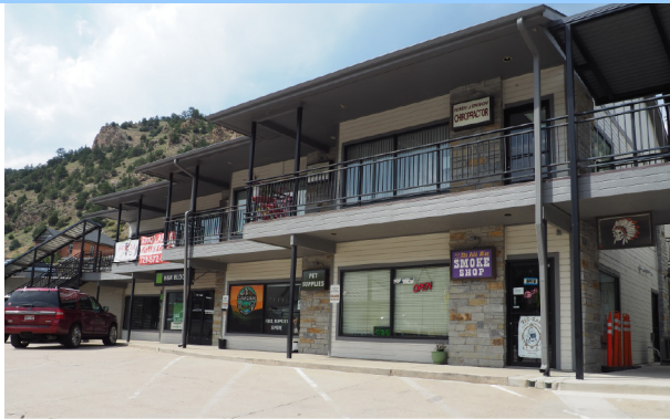
GAO site visit observations in Idaho Springs, Colorado.
