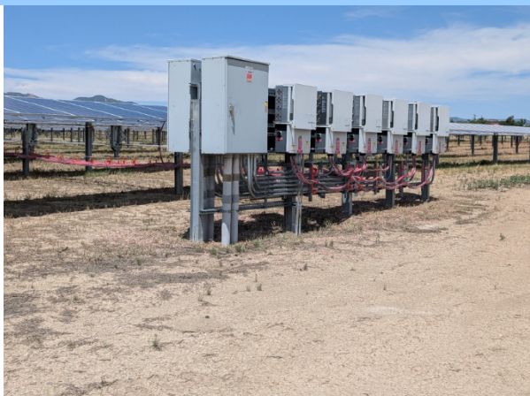
GAO site visit observations in Cañon City, Colorado.
