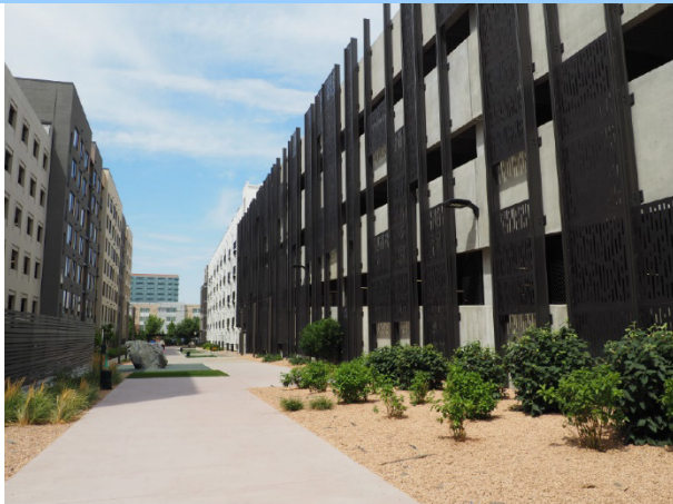
GAO site visit observations in Aurora, Colorado.
