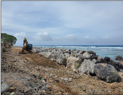
Construction of sea wall.
