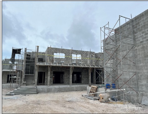
Construction of new classrooms.
