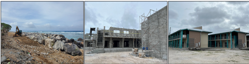
Construction of sea wall.
