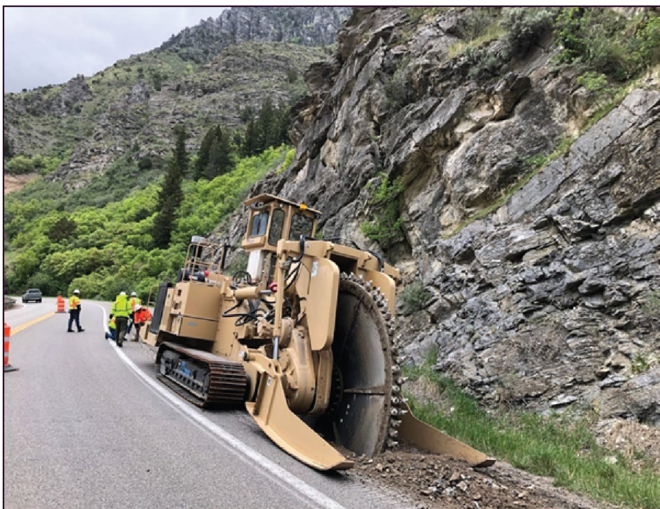
Figure 1: Example of Excavation to Install Fiber Optic Cables in a Federal-Aid Highway Right-of-Way
