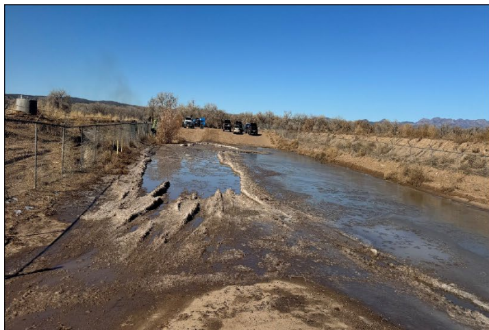
Figure 10: Wastewater Treatment Emergency in Santo Domingo Pueblo
