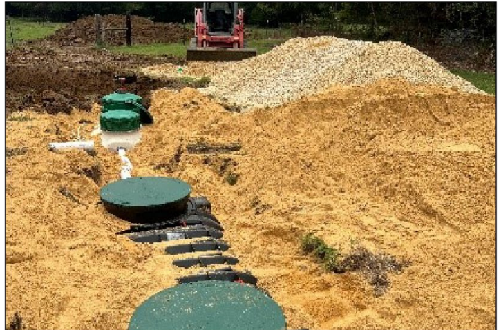
This organization installs advanced wastewater treatment systems for homes where conventional systems would not be appropriate due to poor soil quality or the height of the water table.
