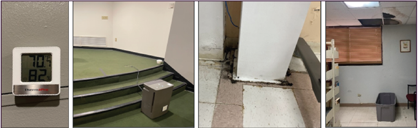
Left: Monitor shows high humidity reading in one Georgia library basement which holds storage. Left/Middle: Portable dehumidifier pictured in same basement. Right/Middle: Mold on second floor of partially operational library in Puerto Rico. Right: Storage bins catch leaking water from ceiling in another library in Puerto Rico.
