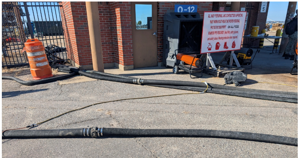
Figure 4: Pier at Naval Station Norfolk, VA Using Temporary Above-Ground Utilities
