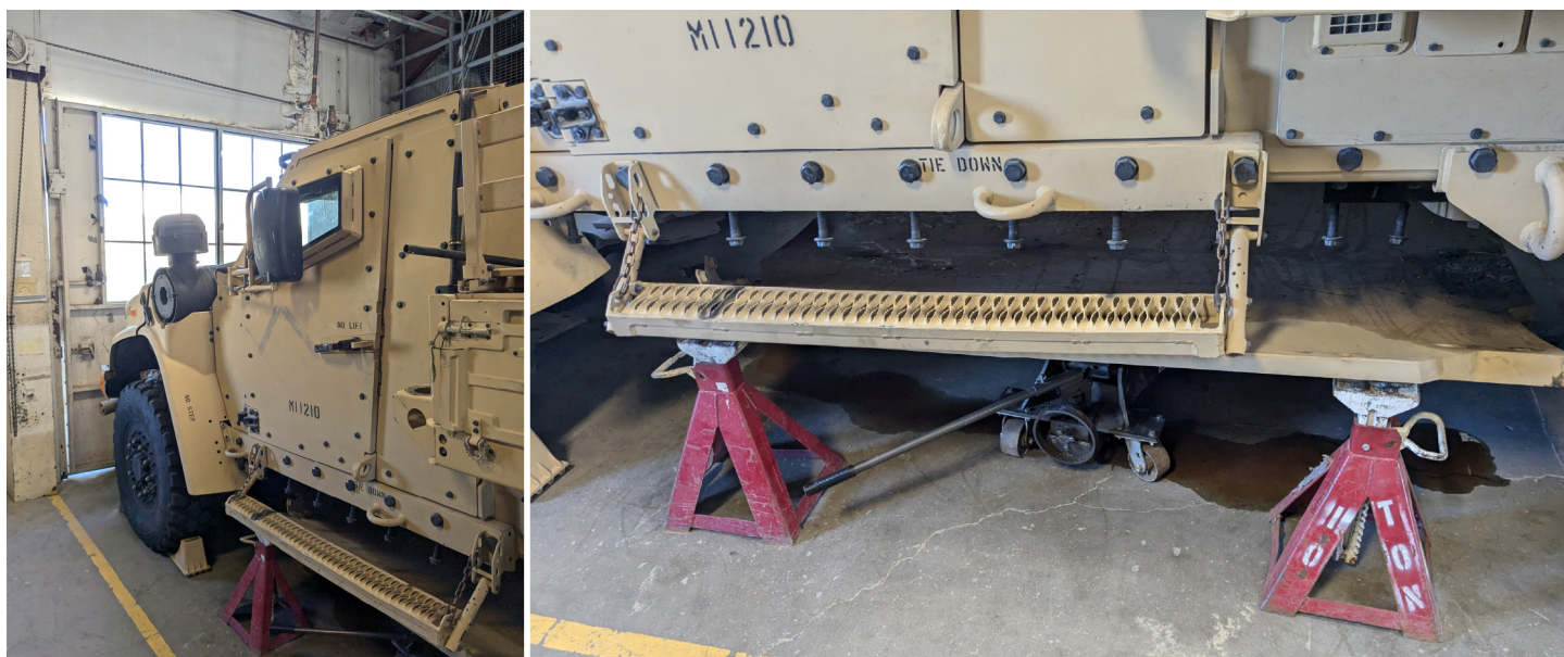
Figure 6: Aging Vehicle Maintenance Facility Planned for Repair at Twentynine Palms Marine Corps Air Ground Combat Center, CA
