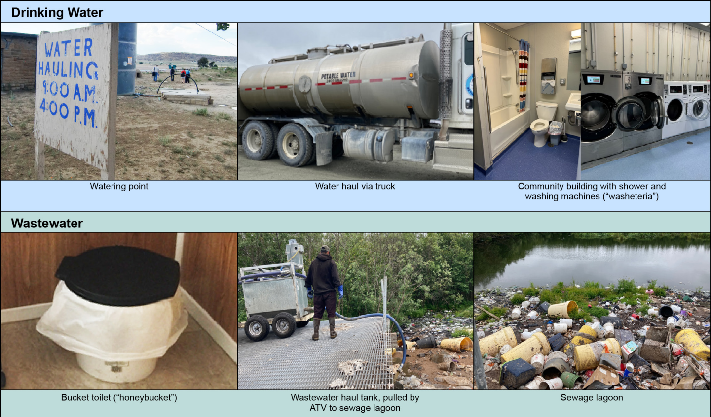
Figure 1: Examples of Drinking Water and Wastewater Systems in Tribal Communities Not Served by Regulated and Centralized Water Systems
