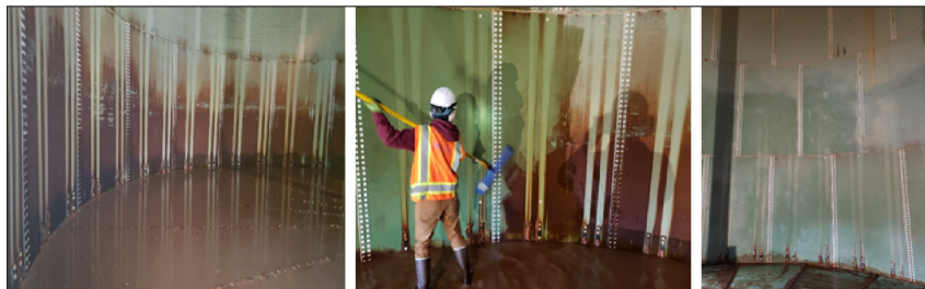
Before water storage tank cleaning Cleaning of tank
