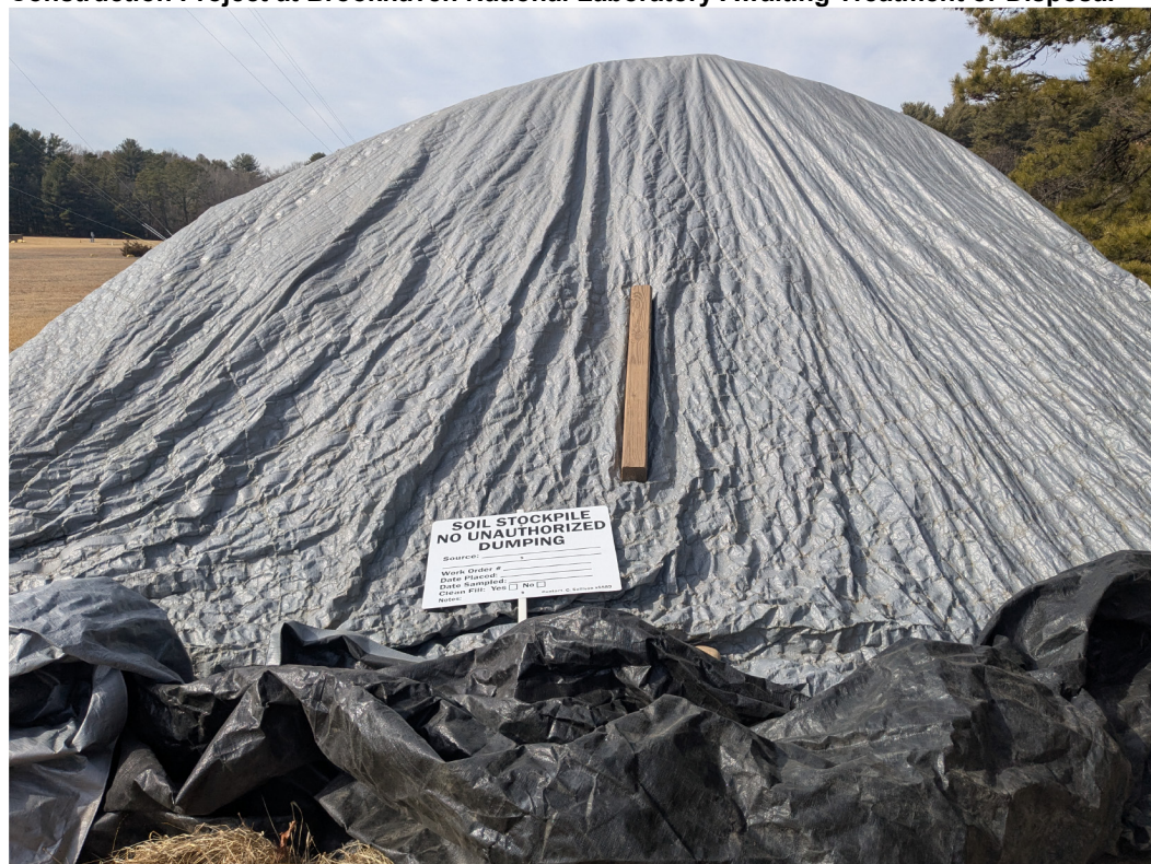
Figure 9: Soil Contaminated with Per- and Polyfluoroalkyl Substances Excavated During a Construction Project at Brookhaven National Laboratory Awaiting Treatment or Disposal
