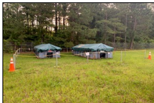
Roll-off containers holding a solidified mixture of AFFF and cement awaiting disposal at the Savannah River Site (SC) .
