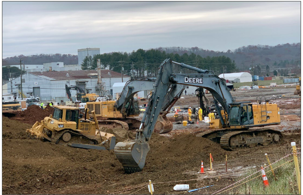
Figure 5: Workers Remove Contaminated Soil from Oak Ridge Office of Environmental Management
