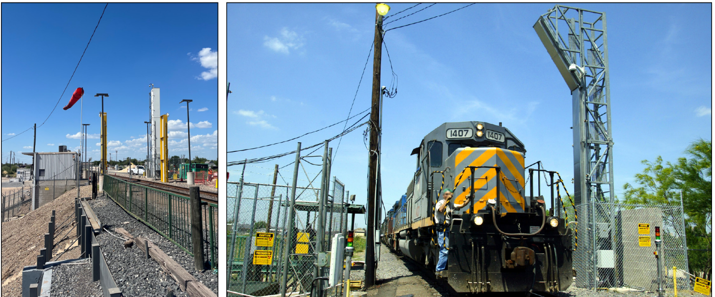
Figure 7: Non-Intrusive Inspection (NII) Rail System in Laredo, Texas (left), and a Train Proceeding Through a NII Rail System (right)
