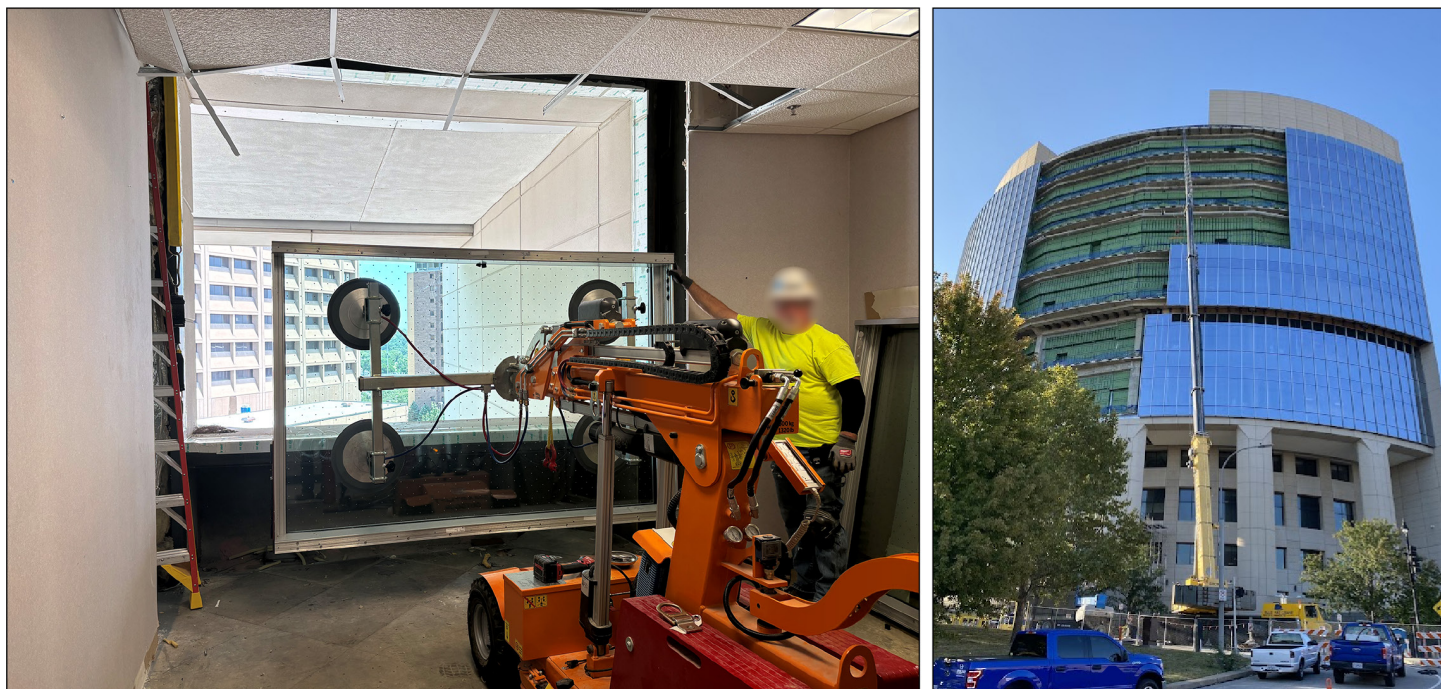
Figure 5: Installation of Low Embodied Carbon Glass Window at Charles E. Whittaker U.S. Courthouse in Kansas City, Missouri, in June 2024
