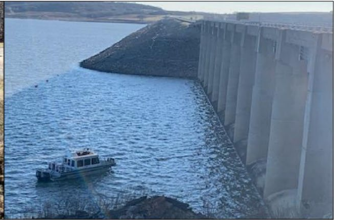
Survey boat conducting a scan to determine location and volume of flood debris, which impacted operations of one of the gates used to regulate water flow.
