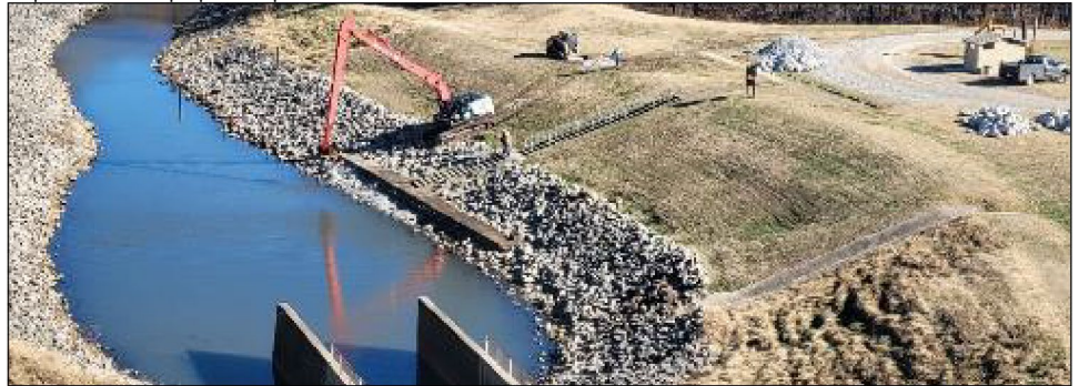
Example of Corps Operations and Maintenance Work Replacement of riprap stone protection on the outlet channel bank.
