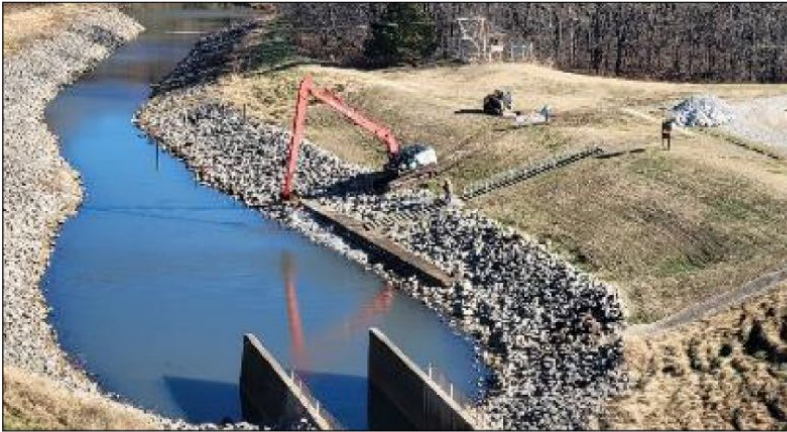
Replacement of riprap stone protection on the outlet channel bank.
