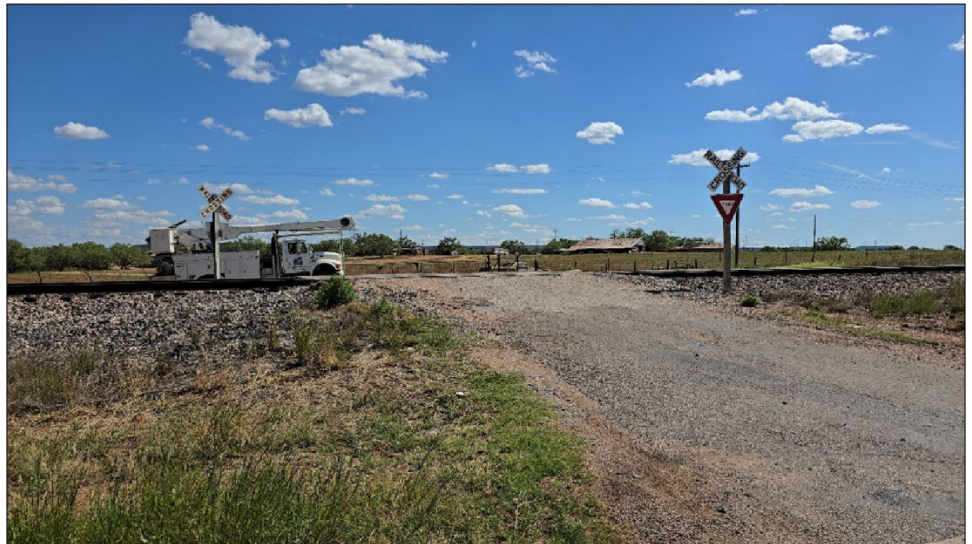
Figure 8: A Humped Grade Crossing in Trent, Texas, Prioritized for Railway-Highway Crossings Program Funded Safety Improvements
