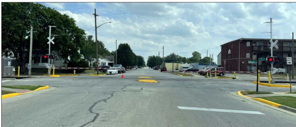
Figure 12: Completed Railway-Highway Crossings Program Project in Seymour, Indiana, That Added Gates and Flashing Lights on the Sides of the Roadway and Medians
