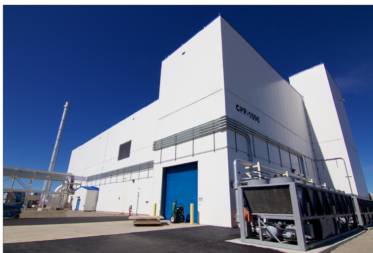
Figure 13: The Integrated Waste Treatment Unit That Was Considered for Treating the Calcine Waste and Currently Treats Sodium-bearing Waste
