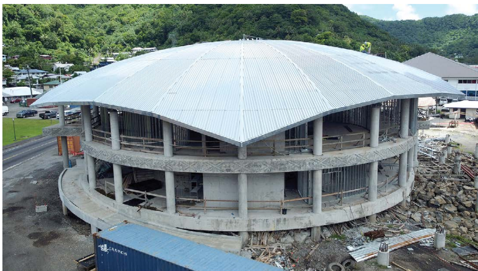
Figure 18: American Samoa Fono Legislature Building, Under Construction
