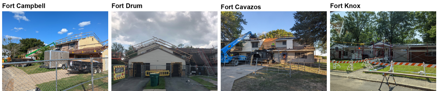
Figure 12: Examples of Integrated Development Plan Roof Replacements
