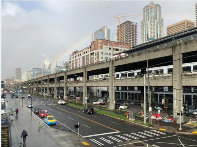
Before: A section of State Route 99, before removal.
