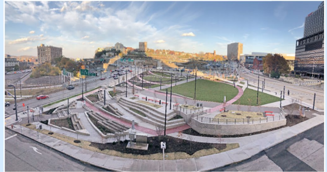
After: The same section of land with a cap park built over Interstate 579.
