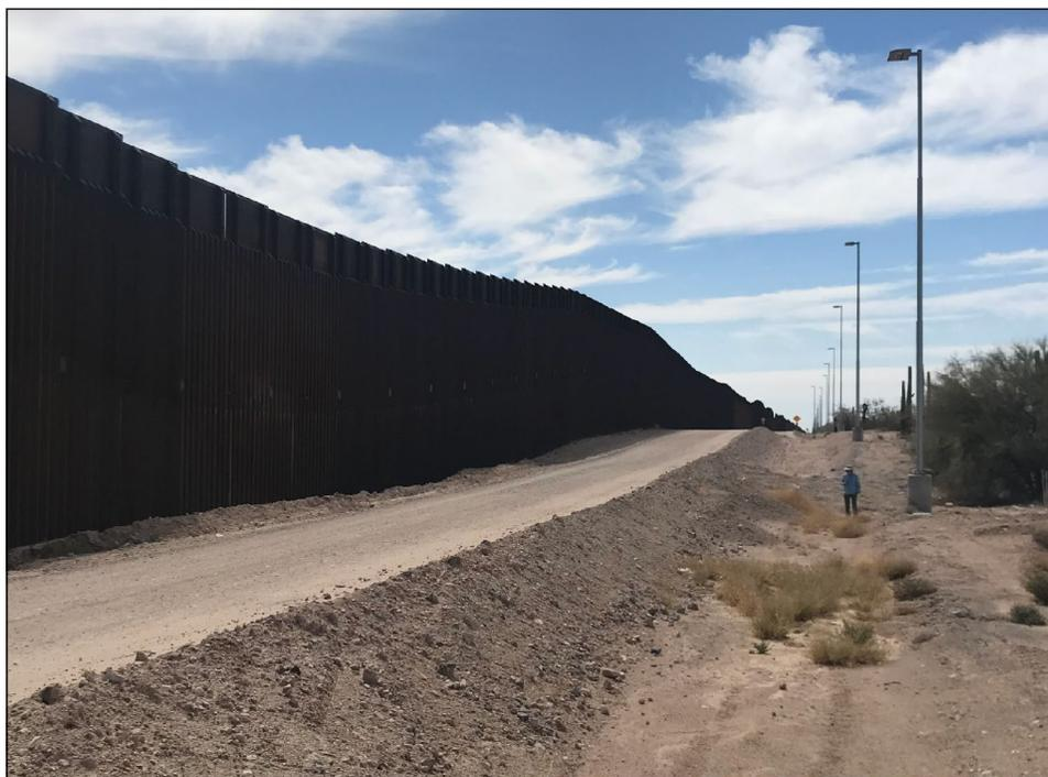
Raised roadbed in Arizona impeding water flow from right side of photo to left (see GAO staff at base of light pole for scale)
