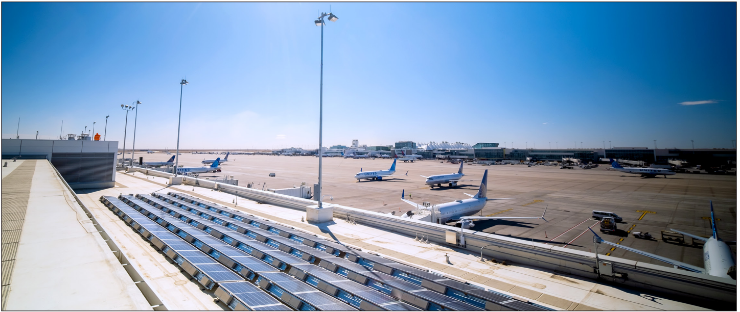
Figure 3: Example of Solar Panels at Denver International Airport
