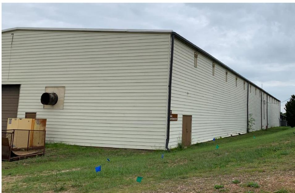
According to an Army official, this World War II-era warehouse is still in use on Fort Leonard Wood, Missouri, although it is difficult to sustain given current funding. The inlet pipe at the front end is for hooking up an external climate control system.
