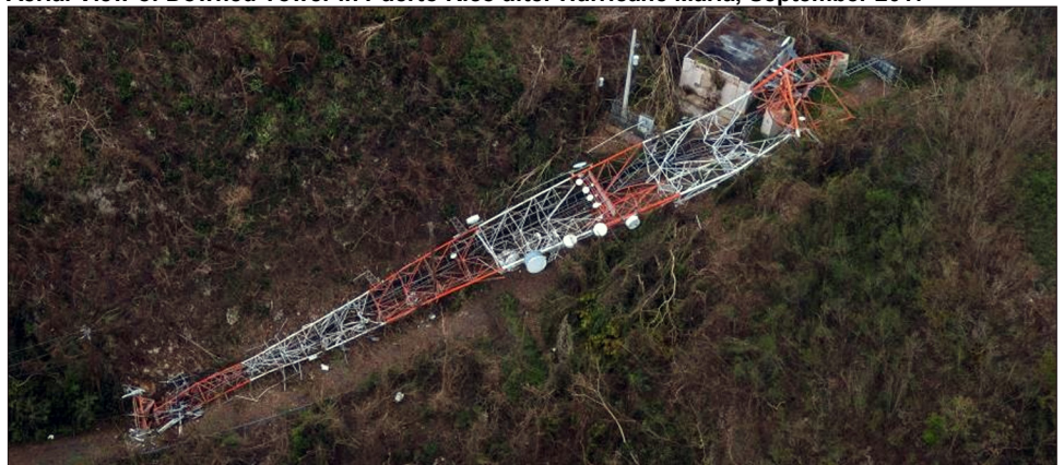
Aerial View of Downed Tower in Puerto Rico after Hurricane Maria, September 2017
