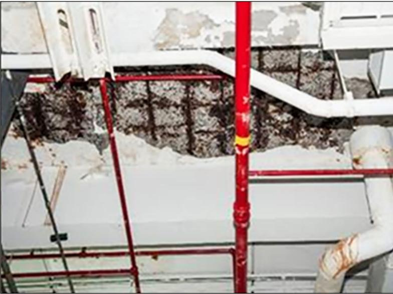
Concrete failure from 2014 on the ceiling, resulting in collapse.
