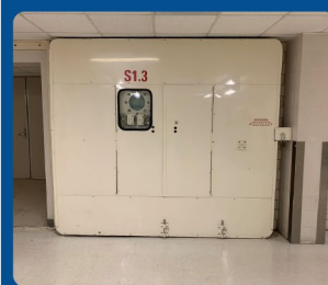
Watertight enclosure to prevent floodwater damage
