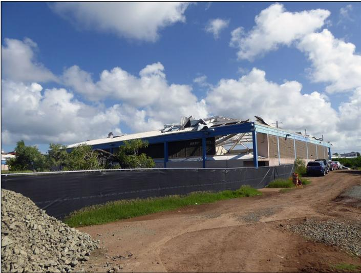
This school building in St. Croix sustained severe hurricane damage, including a collapsed roof.
