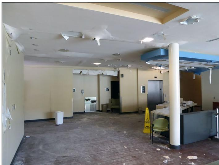
Damage to the hospital's roof allowed water to infiltrate the facility, severely damaging check-in areas, hospital rooms, medical equipment and records, and offices.
