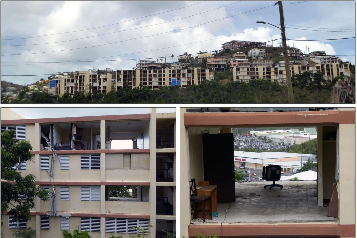
Hurricane force winds and flying debris smashed exterior windows and damaged apartments in a public housing facility in St. Thomas.
