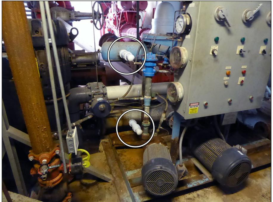
Of the facility's three pumps responsible for providing water to the main hospital building, only one remained operable as of March 2019. Hospital personnel told us they have taken steps to temporarily mitigate the potential for failure, including by installing pipes to relieve pressure.
