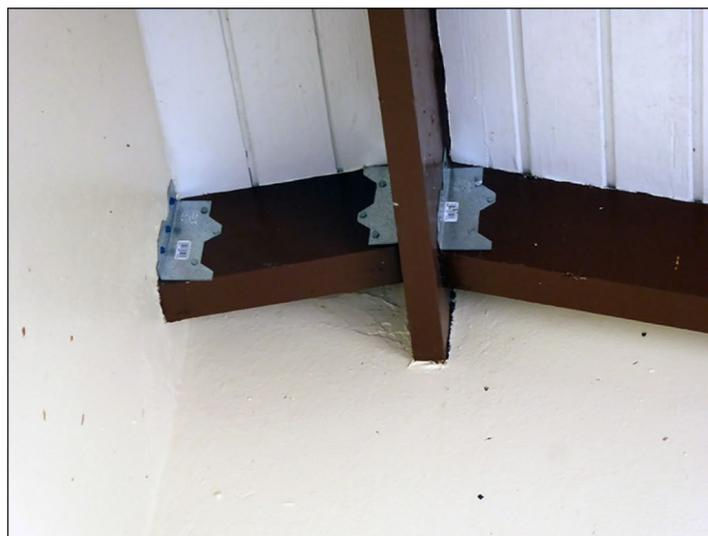
Home with completed permanent roof replacement through Phase II of the STEP pilot program, which included the installation of hurricane clips to increase the roof’s resiliency during hurricane-strength winds.
