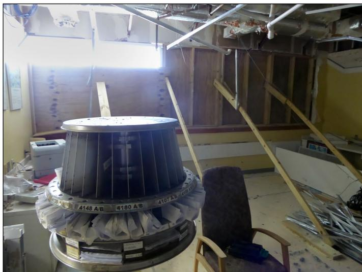
Broken windows caused water and wind damage to a nurses' station. Hospital personnel erected temporary wooden holdings until the station's walls and windows can be repaired.
