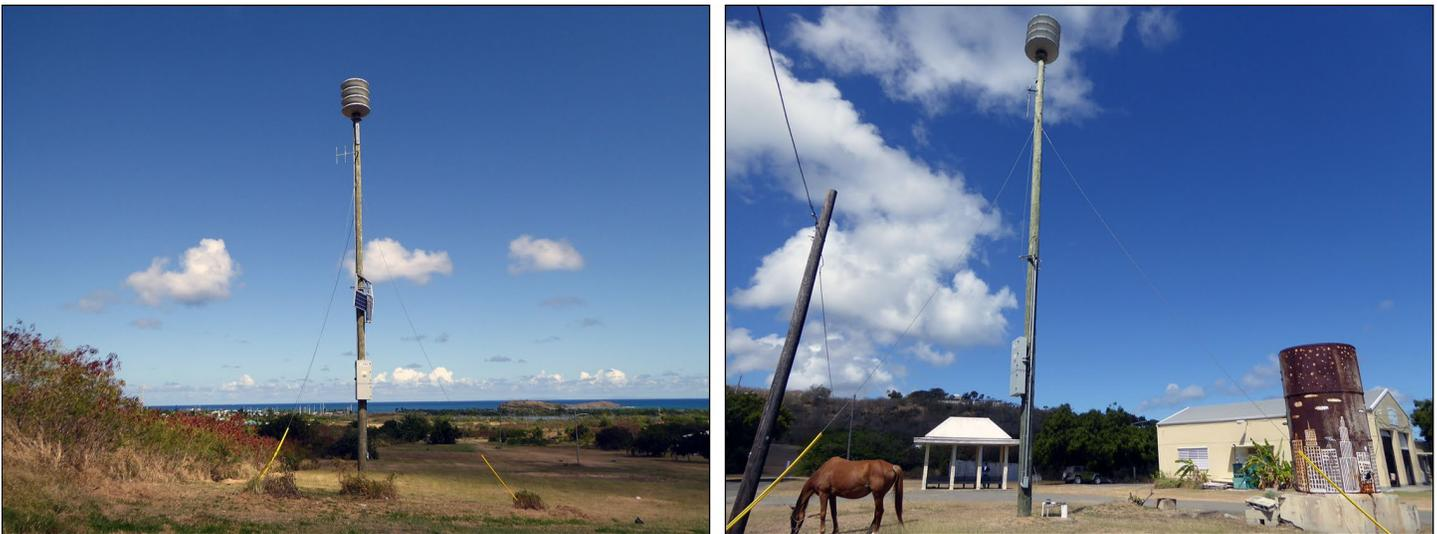
Two tsunami warning system stations in St. Croix, U.S. Virgin Islands. Each station comprises a pole, a siren head to broadcast warnings, a solar panel, stabilizing guy wires, and other ancillary equipment.
