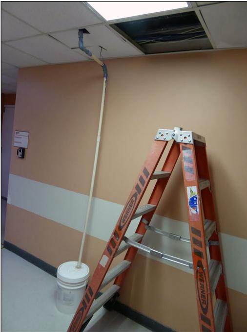
An example of a temporary measure to capture continued water infiltration from the facility's damaged roof.
