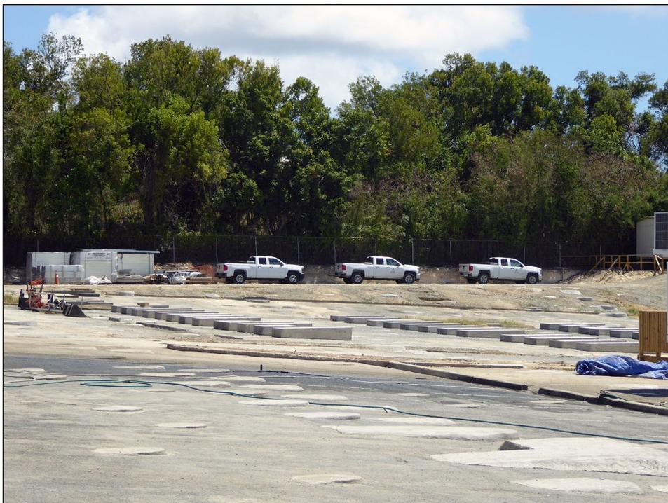
In March 2019, foundations were being constructed in the Governor Juan F. Luis Hospital and Medical Center parking lot to support the installation of modular units. These units will serve as a temporary medical facility until a permanent facility is completed. As of July 2019, the modular units had been erected and contractors were working to complete, among other things, the electrical, plumbing, and heating, ventilation, and air conditioning systems, according to hospital personnel.
