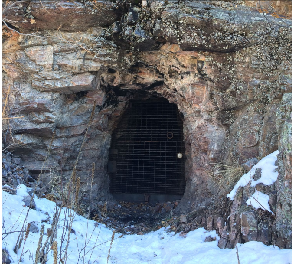
Figure 4: Abandoned Hardrock Mine Tunnel Opening Secured with a Gate to Allow Bat Access on Bureau of Land Management Land in Colorado
