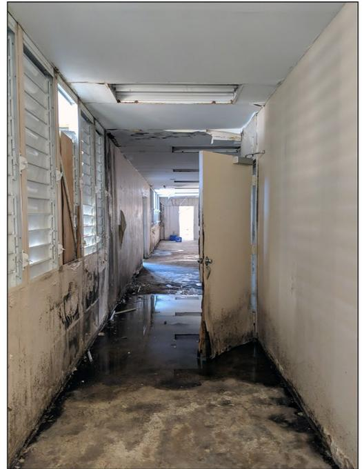
Interior damages to a school in Puerto Rico from water infiltration with standing water and moldy walls.
