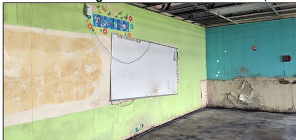
Classroom with mold on floors and water damage on the walls at a school in San Juan, Puerto Rico.
