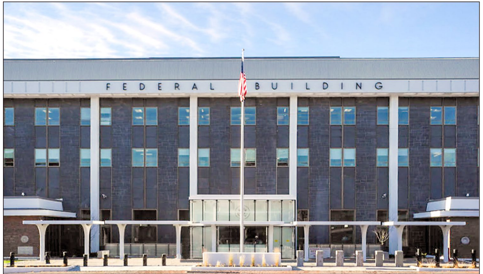
Figure 5: Margaret Chase-Smith Federal Building and Courthouse's Building Exterior with New Entry Pavilion
