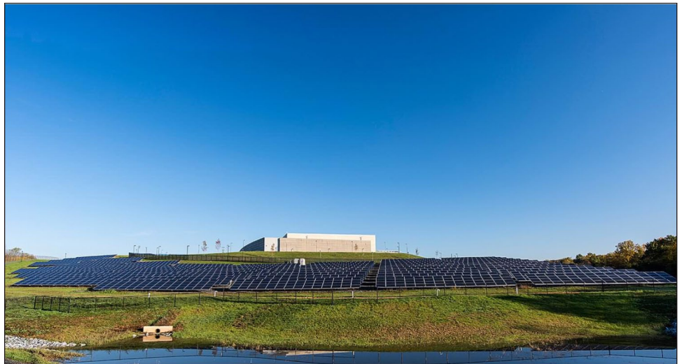
Figure 9: Social Security Administration, National Support Center - On-site Solar Panel Array outside the Data Center
