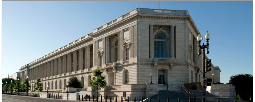
Cannon House Office Building, Washington, D. C.
