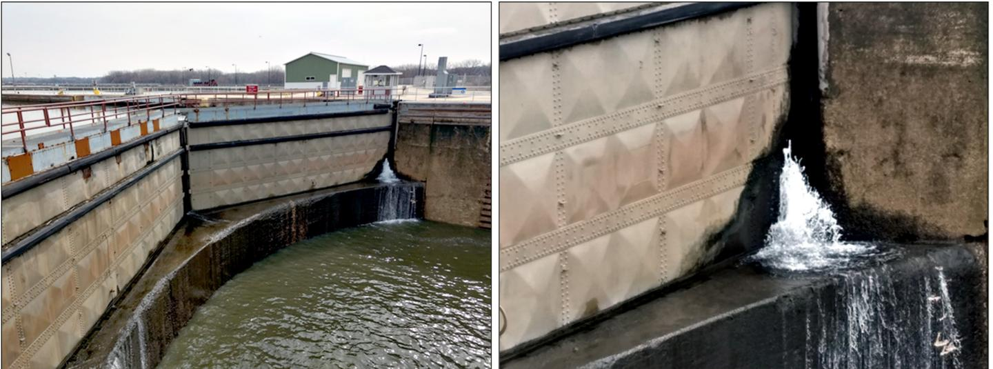
Closed lock gates with water leak in lower right-hand corner, Brandon Road Lock and Dam, Joliet, IL
