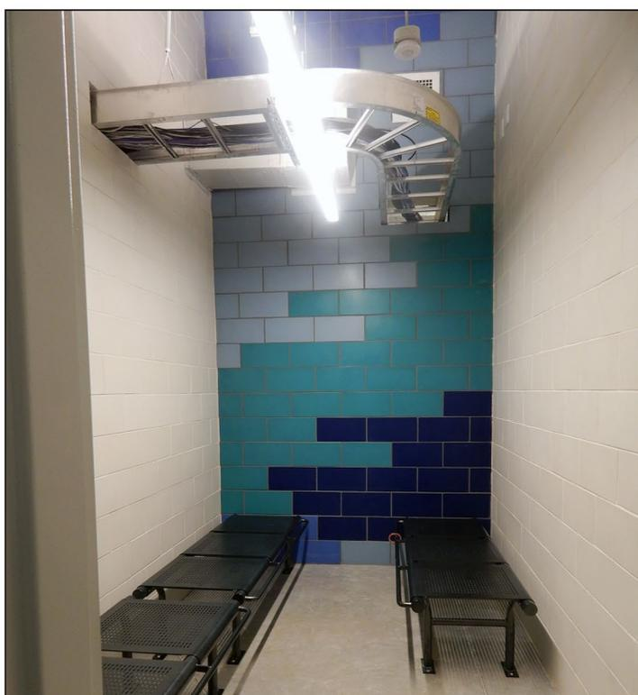
CBP officers identified that exposed cabling accessible to detainees as seen in this photo is a safety hazard at a land border crossing on the southern border.
