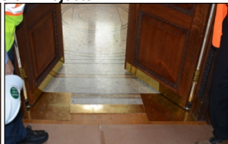
Work at the Library of Congress to reverse the swing of doors to allow for the more orderly evacuation of occupants in the event of an emergency.
