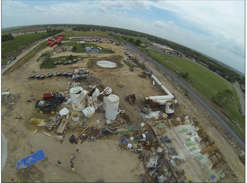
Figure 1: Photographs of Damage from the Explosion in West, Texas in April 2013
