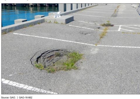
Figure 2: Damaged Dock at Naval Station Norfolk
