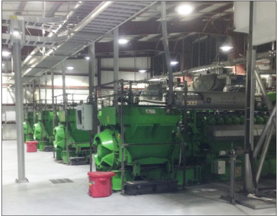
Figure 7: 1.4 Megawatt Generators at Landfill Gas Plant at Joint Base Elmendorf-Richardson, Alaska
