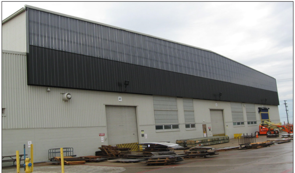
Figure 5: Solar Wall at Letterkenny Army Depot
