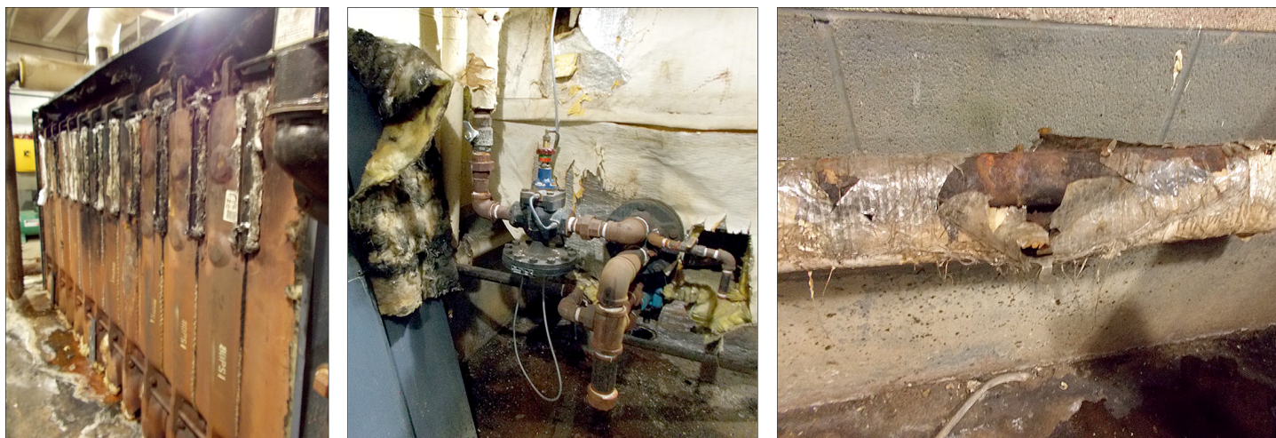
Figure 3: Aging Boiler Systems at a Bureau of Indian Affairs-Operated School Built in 1959
