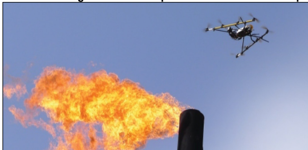
Flare stack inspection
