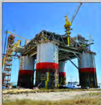
Chevron Corporation's Big Foot tension leg platform undergoing construction; Ingleside, Texas.
